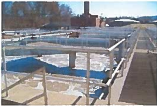
This is a photo of the Northampton Wastewater Treatment Facility.
