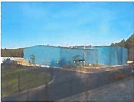
This is a photo of the Northampton Water Treatment Plant.
