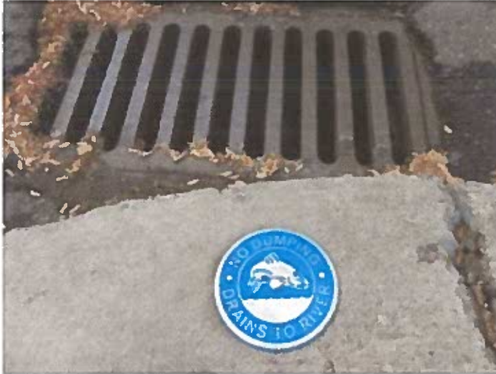
Photo of the top of a catch basin.
